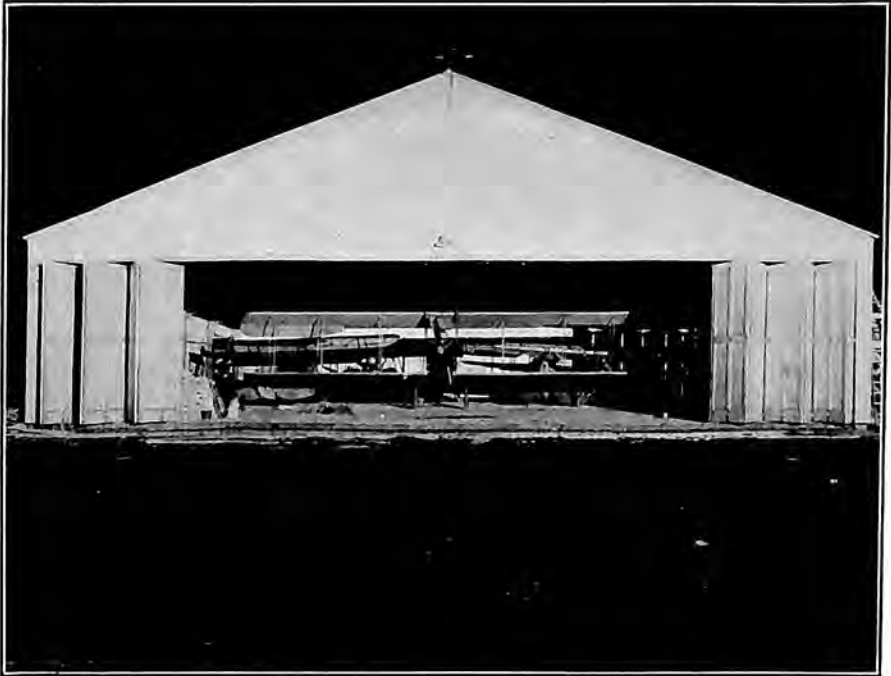
Hangar Illuminated by B. B. T. Lighting Equipment.
