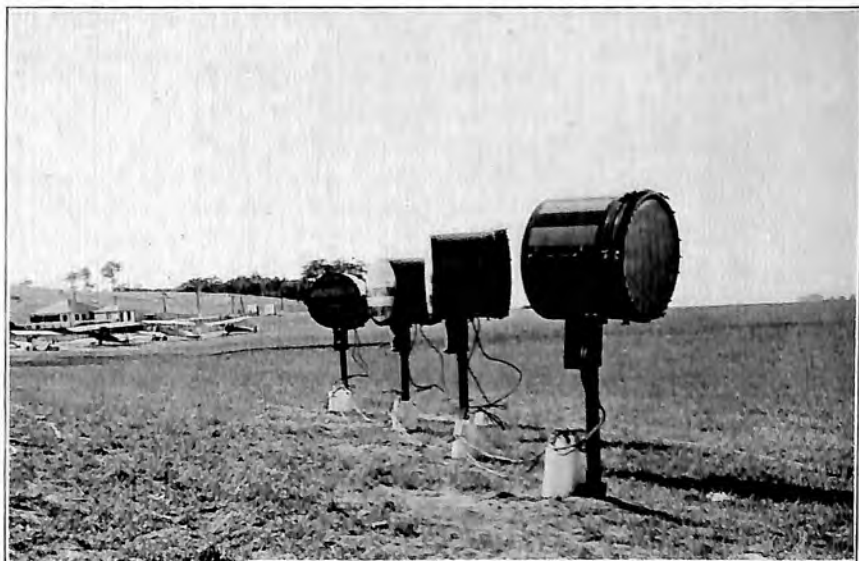
Grouped System of Westinghouse Airport Floodlight Projectors, Bettis Field.
