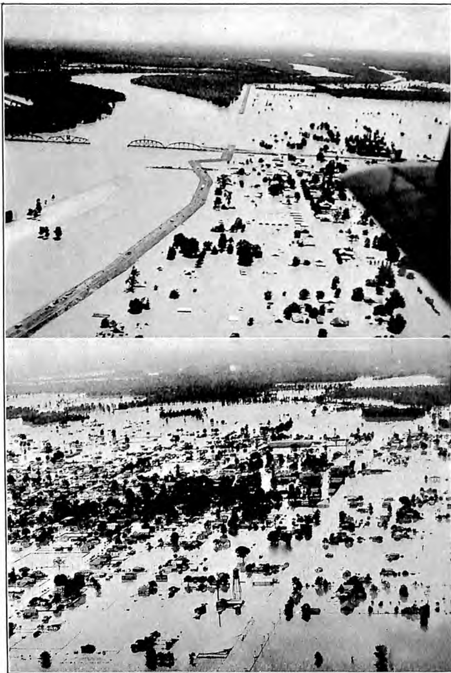
(Top) Melville, La.—Bridge Span Washed Out. (Bottom) Dermott, Ark.—Taken during Flood Periods of May, 1927.—Official Photograph, U. S. Army Air Corps.
