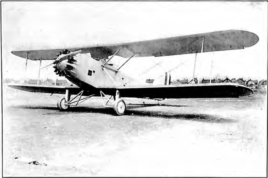
Martin Navy Bomber. Engine, Pratt & Whitney "Hornet."
